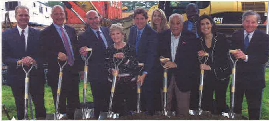
Groundbreaking for St. Regis Residence Rye. From left: Tim Perini, project executive at Alfred Weissman Real Estate; Jeffrey Greenberg, principal at Heritage Capital Group; Scott Rechler, CEO of RXR Realty; Connie Weissman; Alan Weissman, principal of Alfred Weissman Real Estate; Gigi Weissman; Angelo Martinelli; Ken Jenkins, Westchester deputy county executive; Dana Jacobsohn, VP of mixed-use development at Marriott International; and Steve Otis, state assemblyman.
